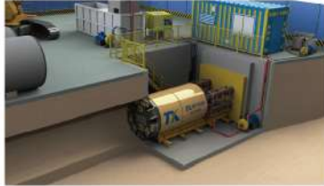
安装顶管机主机 Installation, connection and debugging of pipe jacking machine
