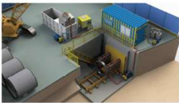
安装始发井内组件 Install auxiliary equipment in starting shaft
